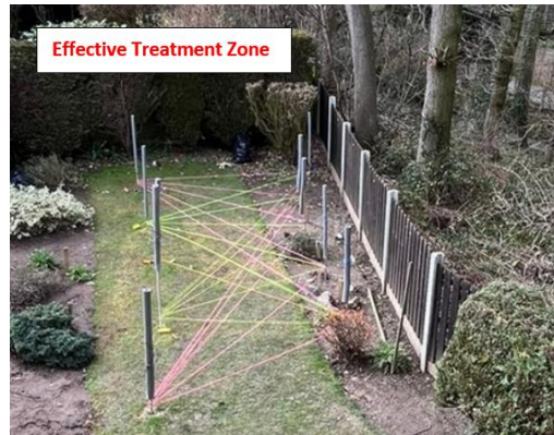
Above, left, electrode array between the house and the trees. Lime is added to the soil to reduce the shrink/swell potential, reduce root activity and moisture change. Below, distortion of building footprint prior to treatment.
