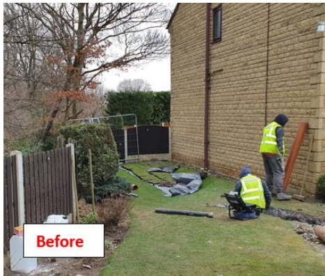
Above, left, electrode array between the house and the trees. Lime is added to the soil to reduce the shrink/swell potential, reduce root activity and moisture change. Below, distortion of building footprint prior to treatment.
